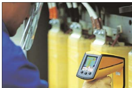
Transformer inspection
